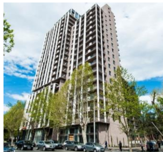
Apartment building: Kazbegi avenue Completion status: 100%
