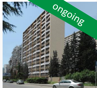
Apartment building: Kartoza Street Completion status: 45% Construction start date: Nov 15
