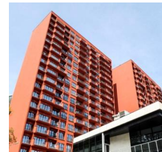
Apartment building: Tamarashvili Street II Completion status: 100%
