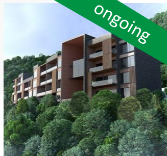
Apartment building: Skyline Completion status: 85% Construction start date: Dec 15
