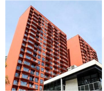
Apartment building: Tamarashvili Street II Completion status: 100%
