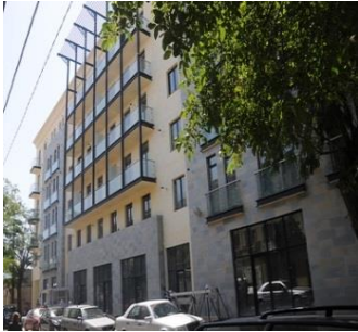
Apartment building: Chubinashvili street Completion status: 100%
