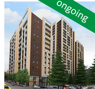
Apartment building: Kazbegi avenue II Completion status: 6% Construction start date: Jun 16
