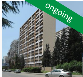
Apartment building: Kartozia Street Completion status: 29% Construction start date: Nov 15
