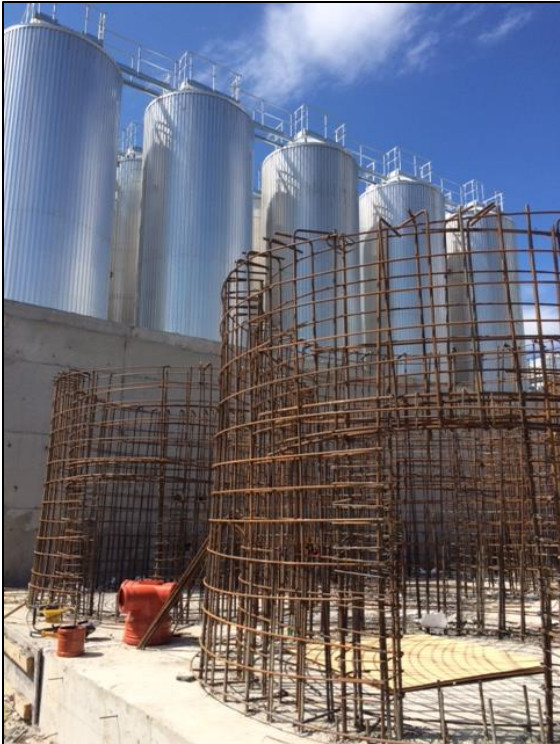
Picture 1: Large container construction site
